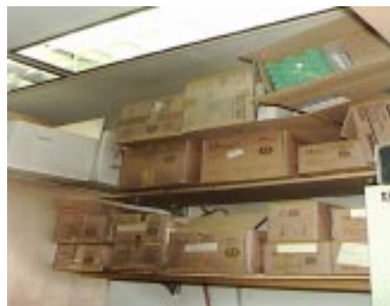
Smoke damage to combustibles stored above waterbath
